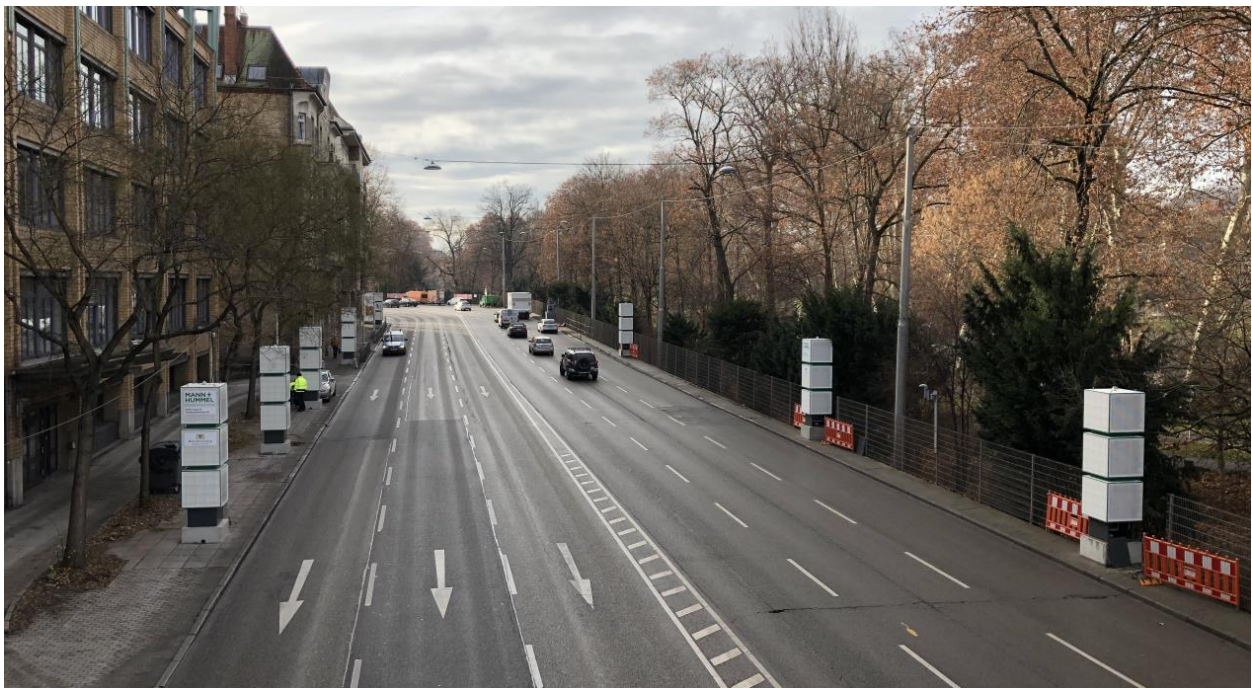
Figure 2.5 – View of the western section of the pilot project following installation of the Filter Cubes (generation 1).
