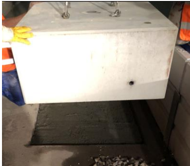
Figure 2.4 – Installation of the foundations.
