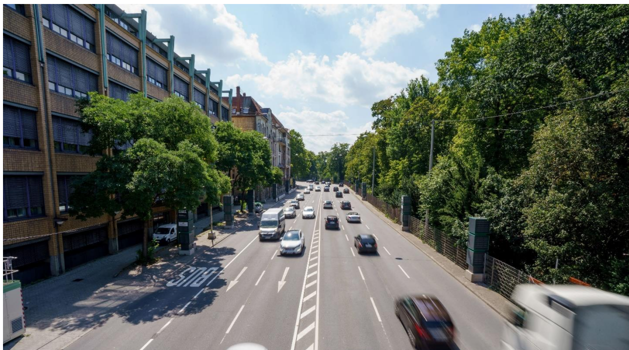
Figure 2.9 – View of the eastern section of the pilot project following installation of the Filter Cubes (generation 2).
