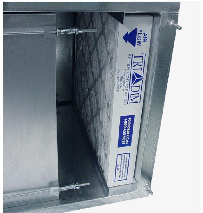
A prefilter installed in the Tri-Lock SB housing.
